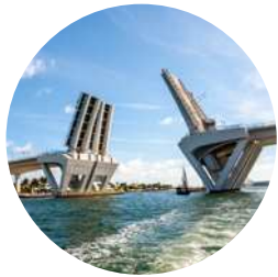
BRIDGES & MOVABLE STRUCTURES
